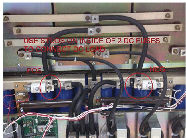
Figure 6: 3060-MS Bus Bar Connections
